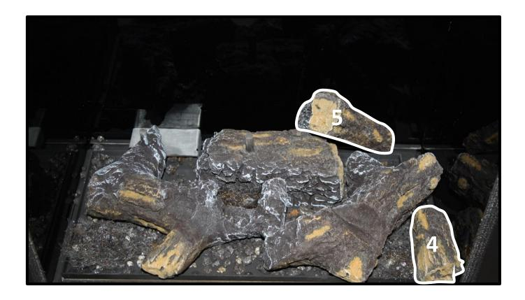
Place a further 2 log shapes as highlighted above. Log No.5 is a Y shaped log.
